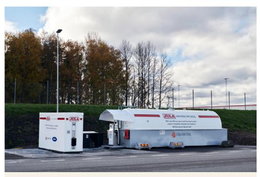
A fuel station for HVO (hydrogenerated vegetable oil) at Jula's warehouse in Skara, Sweden.
