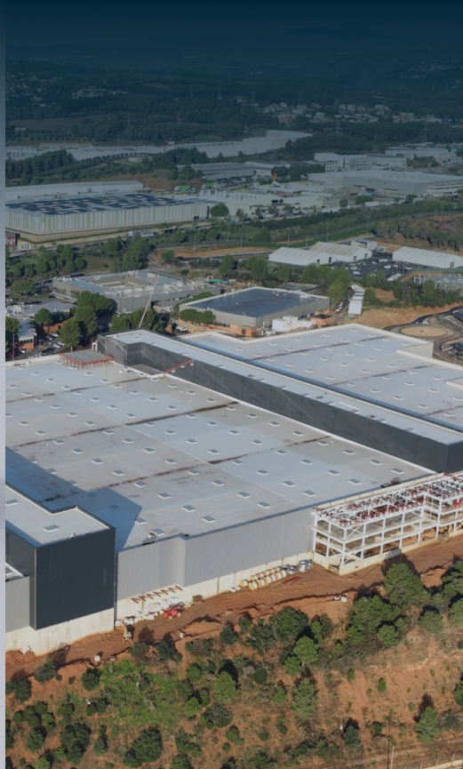
Ramp-up factories for Battery cell and system
